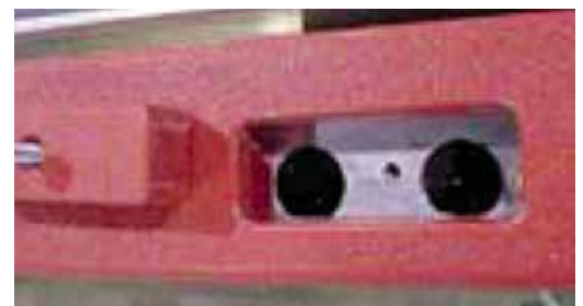
Access panel on topsill allows the glass to be easily adjusted so it stands straight and true without shims.
