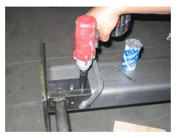
Lift the bottom crossbar into place and fasten. The bottom crossbar is provided as a spacer to help align the towers top and bottom. Make sure to measure between the towers top and bottom to ensure that the top and bottom measurements match.
