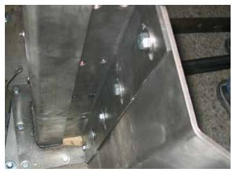
Move frame jambs and threshold into opening and fasten them to the floor and each other.
