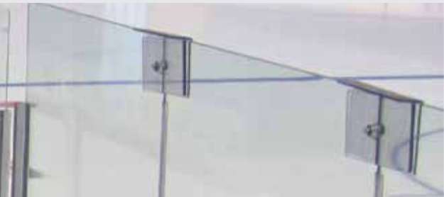
Clips allow each piece of glass to move independently upon impact, maximizing overall flexibility.
